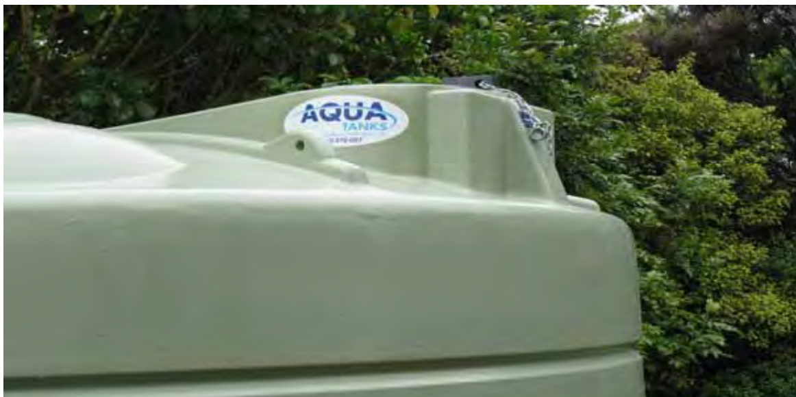
Figure 1: Emergency rainwater tank with locked access cover at Pukerua Bay School
