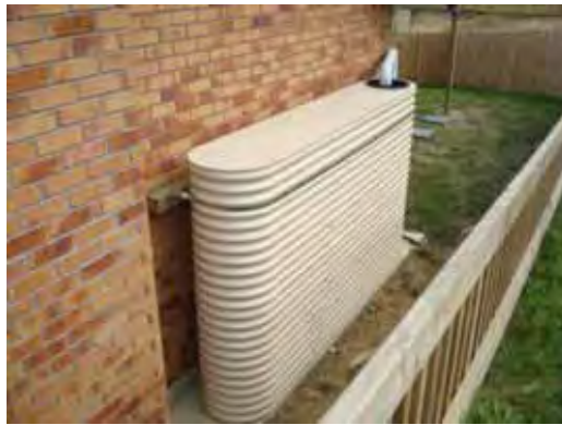
Figure 10: A seismically restrained 1,000 litre rainwater at a dwelling in the North Shore
