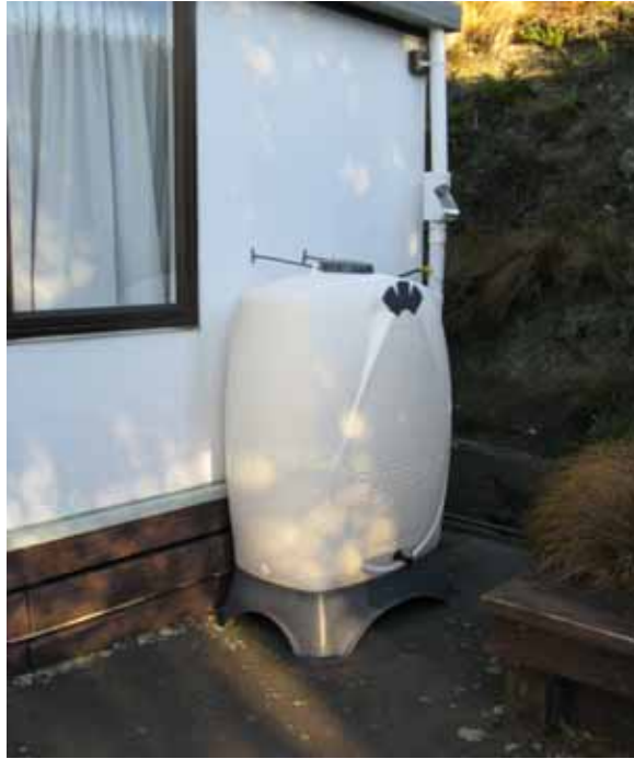
Figure 4: A 600 litre rainwater tank with screened rain head and down pipe water collector at Wellington East Girls College
